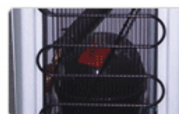
Hermetically sealed reciprocating Compressor
