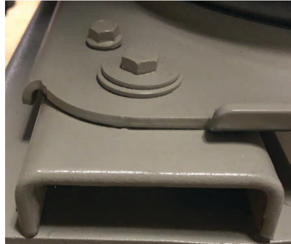
Figure 2: Compressor Base Plate Mounting
