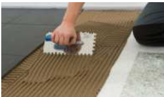
Fig. 3: Number of notches on the tile adhesive comb/trowel depends on the tile size: · 8-notch trowel for tiles from 10x10 cm to 30x30 cm · 10-notch trowel for tiles up to 60 cm x 40 cm
