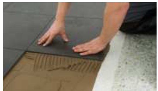
Fig. 6: Press tiles down firmly eliminating any air trapped in the process. Ensure that the depth of the bed is at least 4 mm.
