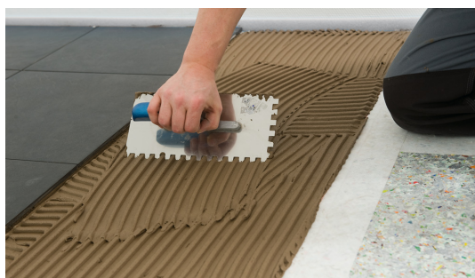
Fig. 3: Number of notches on the tile adhesive comb/trowel depends on the tile size: · 8-notch trowel for tiles from 10x10 cm to 30x30 cm · 10-notch trowel for tiles up to 60 cm x 40 cm
