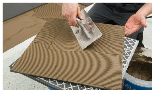
Fig. 4: Also fully apply tile adhesive to the back of the tile.
