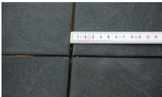
Fig. 7: Observe the grout width: · tiles up 30 x 30 cm have 3 mm minimum grout · 40 x 60 cm tiles will have at least 5 mm grout
