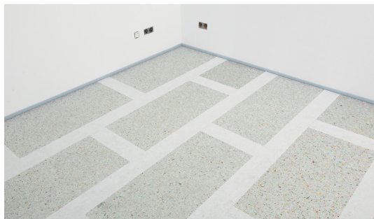
Fig. 1: Install the Strongboard panels evenly on top of the heat panels leaving no air voids.
