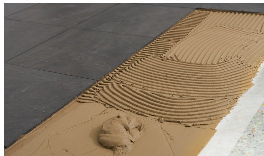
Fig. 2: Prepare the Mapei Elastorapid tile adhesive and apply it to the strongboard.
