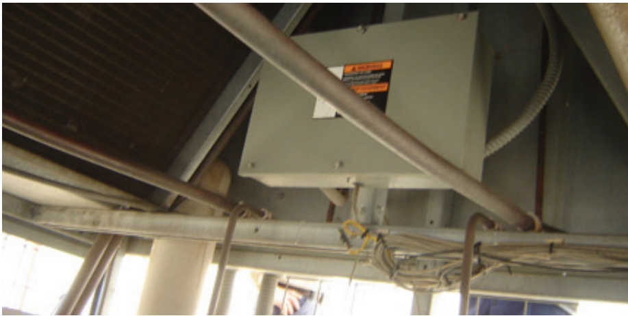
Figure 3. Original drive installation
