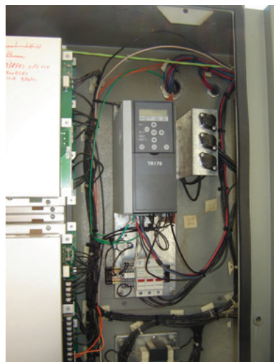
Figure 6. Mounted drive assembly
