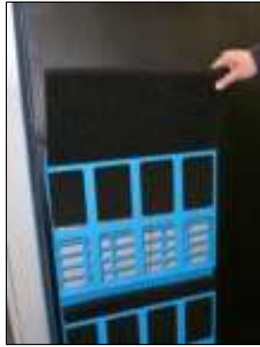
Figure 6-2 Air Pre-Filters Removal
