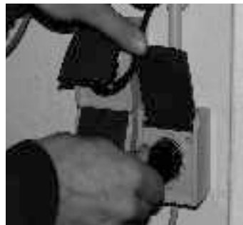
6. Insert cable of pump motor into socket
