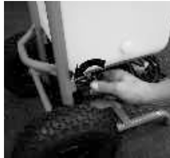
2. Fill tank and open ball valve
