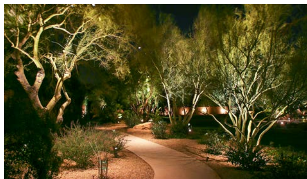
Cross-light mature trees with multiple fixtures to illuminate the full canopy at night.
