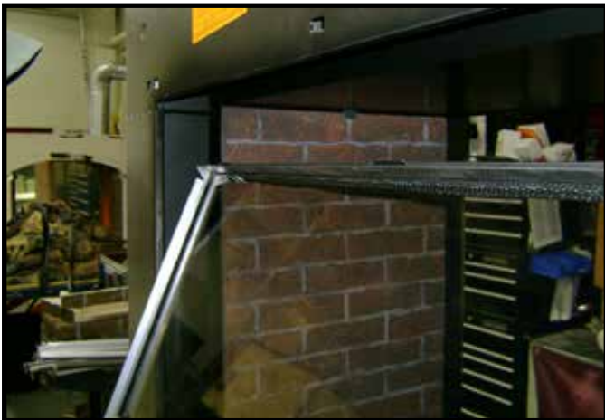
Figure 11.2 Initial Positioning of Frame into Opening.
