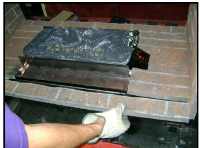
Figure 11.19 Positioning Outer Bottom Refractory.
