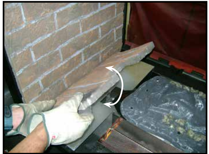
Figure 11.17 Positioning Inner Bottom Refractory
