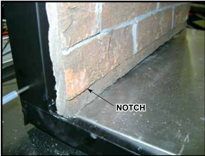
Figure 11.15 Notched End of Side Refractory
