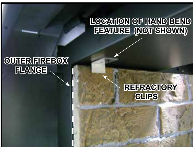
Figure 11.16 Refractory Clip Installation
