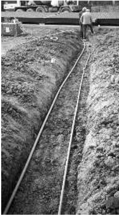
Figure 3-1. Conduit Run in Trench
