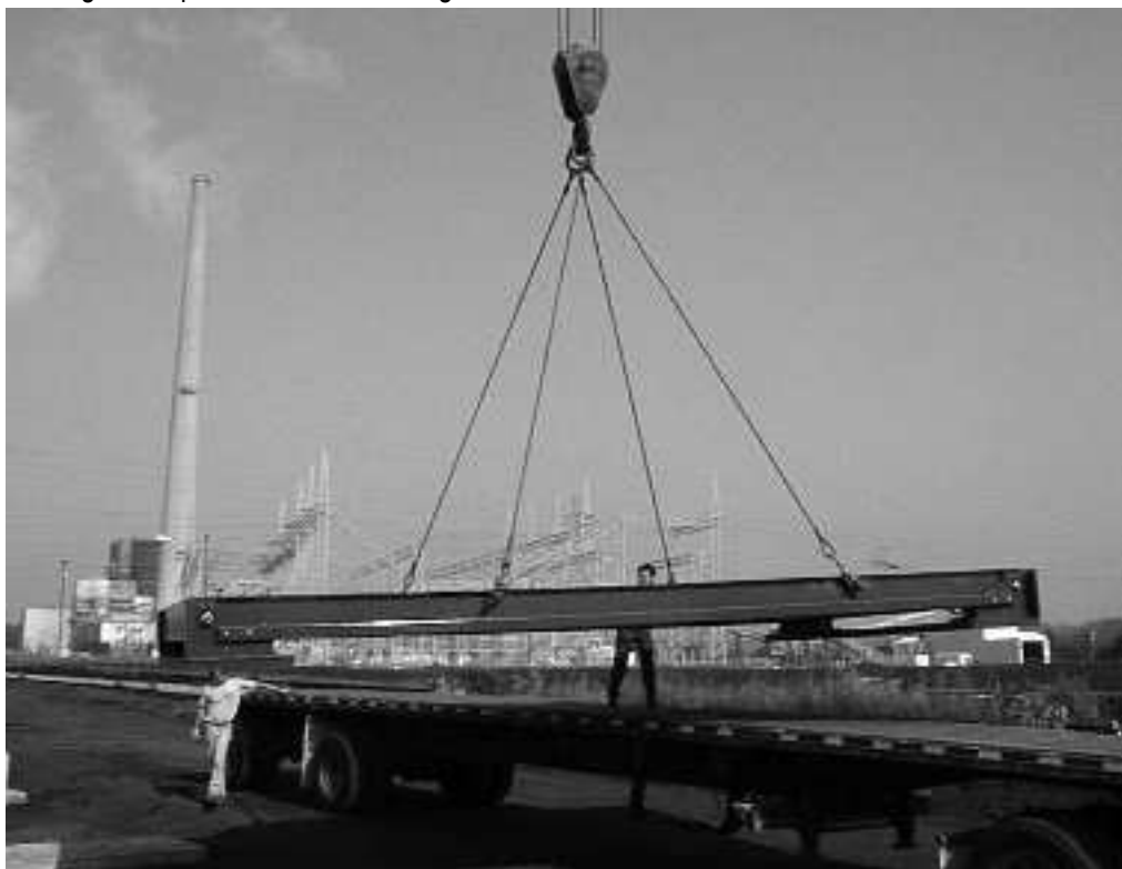
Figure 1-2. Unloading Modules From Truck
