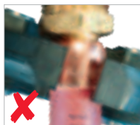
Jaw not square on the crimp ring
