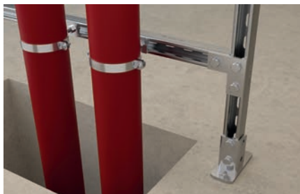
Waste water pipe
