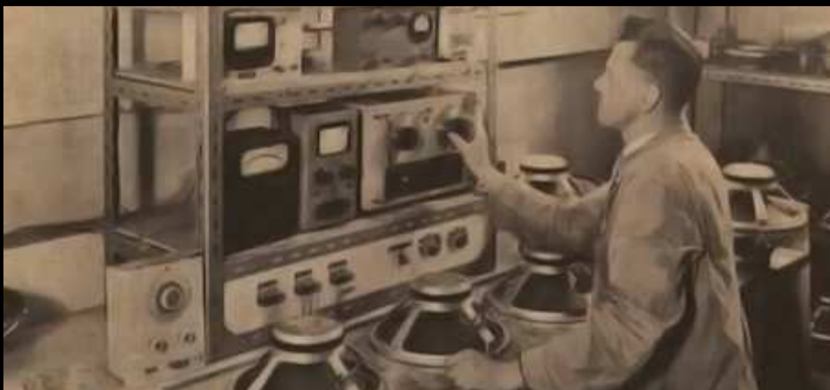
As it was then and so it is now, every Wharfedale speaker is expertly tested over its full frequency range and the bass resonance is checked and noted in the daily production records.
