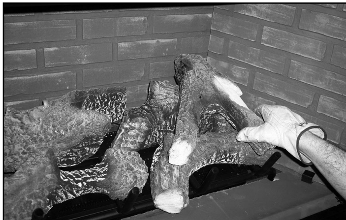
Figure 12.2 Placing Right Top Log
