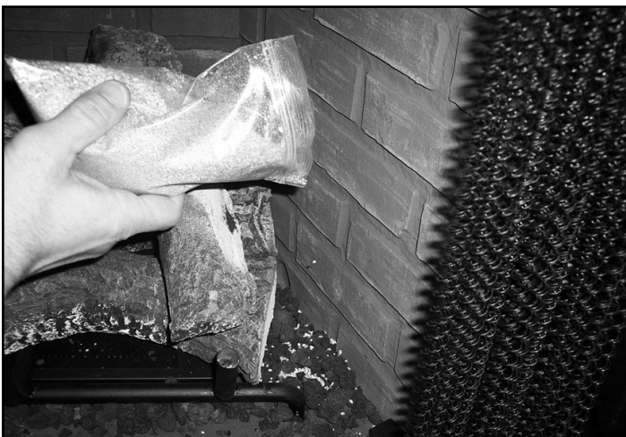
Figure 12.5 Placement of Vermiculite
