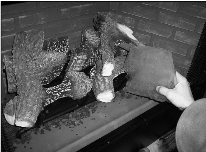
Figure 12.4 Placement of Lava Rock
