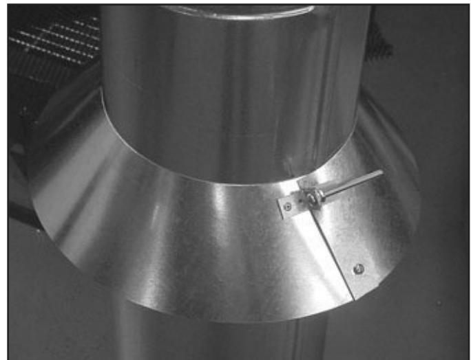
Figure 25 Insert Bolt into Brackets
