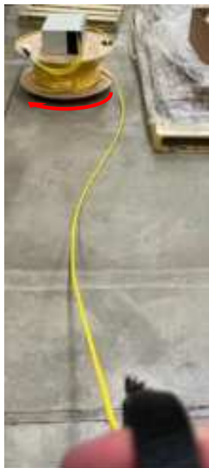
Unspooling with pulling eye
