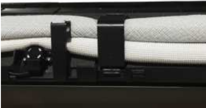
Figure 27: L-bracket Closed (Appearances Will Vary Depending on Indoor Unit Model).
