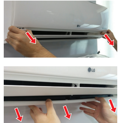
Figure 45: Removing the Bottom Cover, Alternate View.
