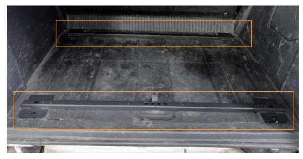
Secure the main body to the mounting brackets  $\ensuremath{\mathsf{D}}$  and  $\ensuremath{\mathsf{E}}.$  Tighten the hardware.
