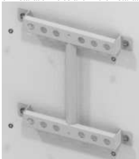
Figure 8: Punch installation holes and fix the installation bracket
