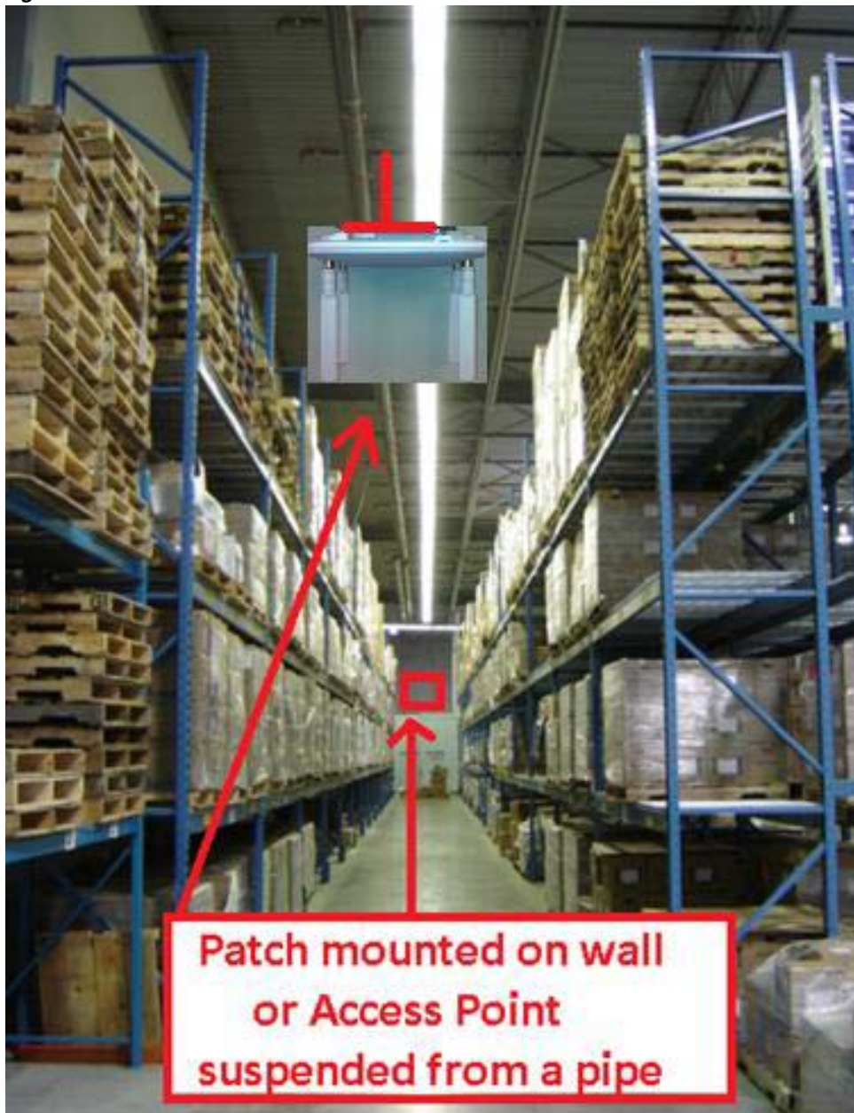
Figure 25 AP Placement in a Warehouse Environment
