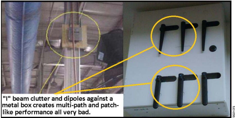
Figure 90 Example of an AP Installation Near Metal and Clutter (Again, Try to Avoid Metal and Clutter)
