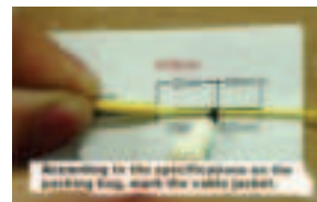
Using the label, measure from the end of the buffer and make a mark between the 250 \mu m and 125 \mu m section
