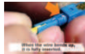
Insert the fiber into the connector body until the strand meets resistance and bows slightly
