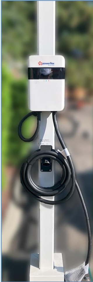
An installed Liteon 48 EV charger on a pedestal
