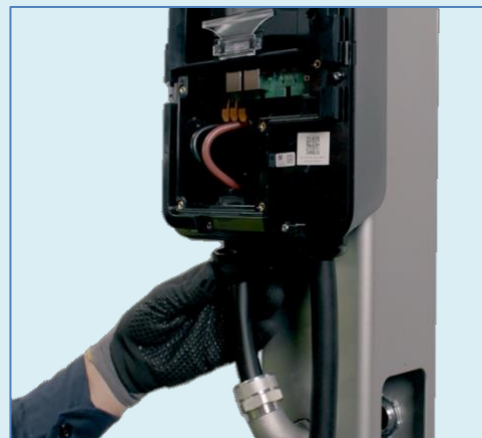
Connecting wiring from the pedestal to the charger
