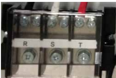
Measure Input Voltage.
