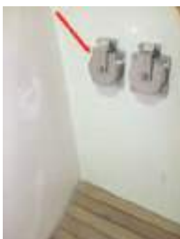
Shore power socket 220V - 32A (Reference 1)
