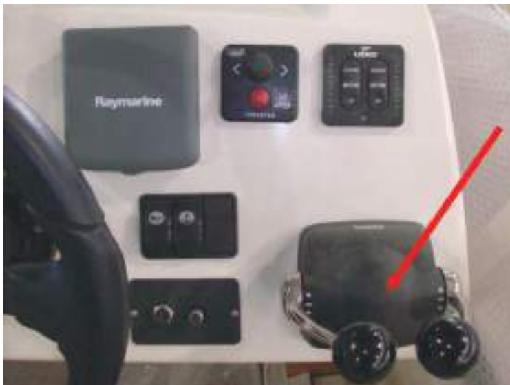
Wheelhouse Flying bridge
