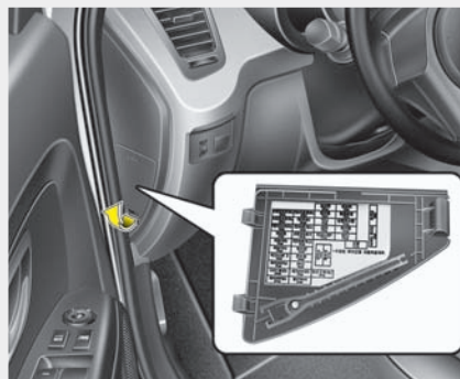
Inner fuse panel
