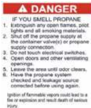
Propane System Label
