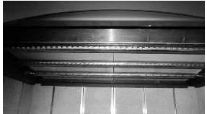
Figure 4.8 Reinstall Baffle Boards
