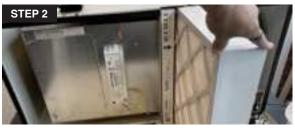
2. After opening the unit's access door, grasps both edges of the HEPA filter and pull with equal force to slide it out.
