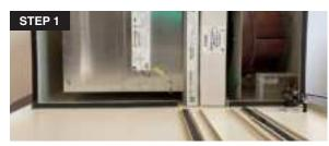
1. Open the filters and motor access door at the front of the unit. Start by unlocking the access door latches.
