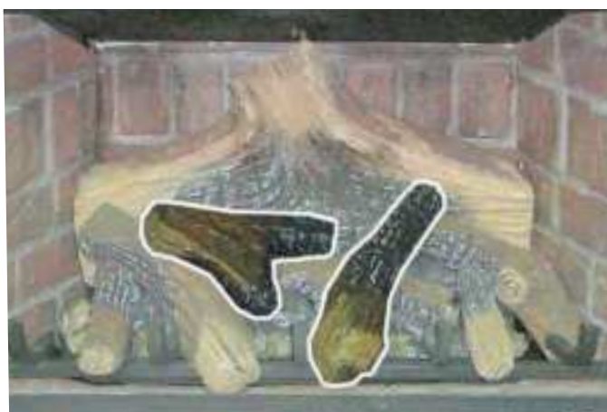
Figure 65: Seventh Stage Log Set Installation.
