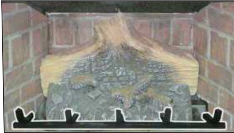
Figure 61: Third Stage Log Set Installation.
