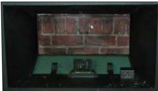
Figure 56: Remove the rear brick panel by pulling it forward off of the ledge.
