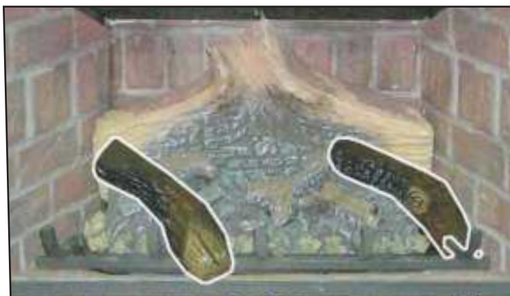
Figure 63: Fifth Stage Log Set Installation.
