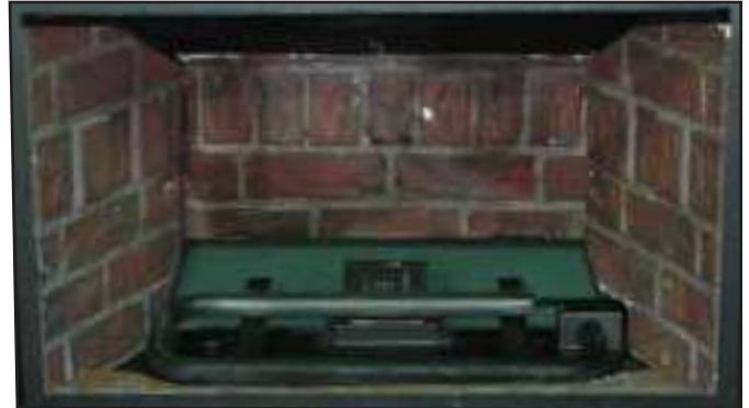
Figure 53: Carefully remove the front brick panel on the bottom of the firebox by lifting it up.
