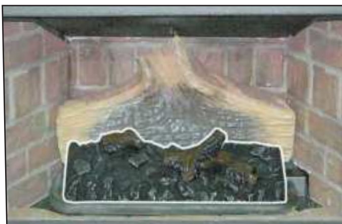
Figure 60: Second Stage Log Set Installation.
