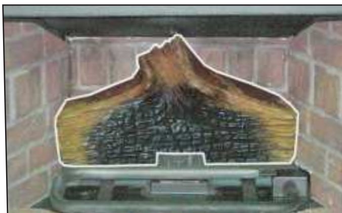
Figure 59: First Stage Log Set Installation.
