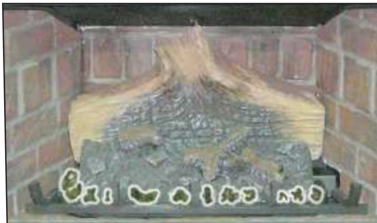
Figure 62: Fourth Stage Log Set Installation.
