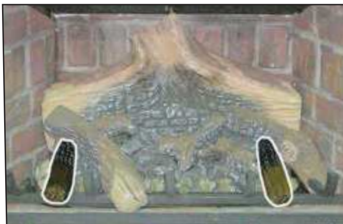
Figure 64: Sixth Stage Log Set Installation.
