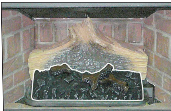
Figure 60: Second Stage Log Set Installation.
