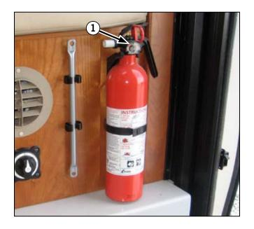
Check the pressure indicator on your fire extinguisher periodically. If it loses pressure, the dry chemical cannot be discharged effectively.
