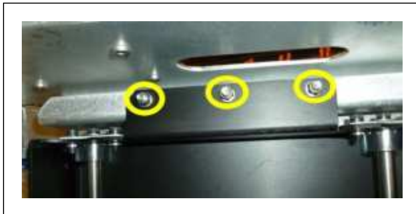
Figure 8-15. Mounting Studs and Nuts at top of Drive Assembly
