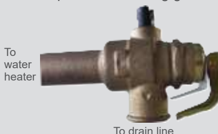
How to operate the easing gear
