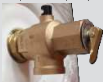
TPR position - top of cylinder
