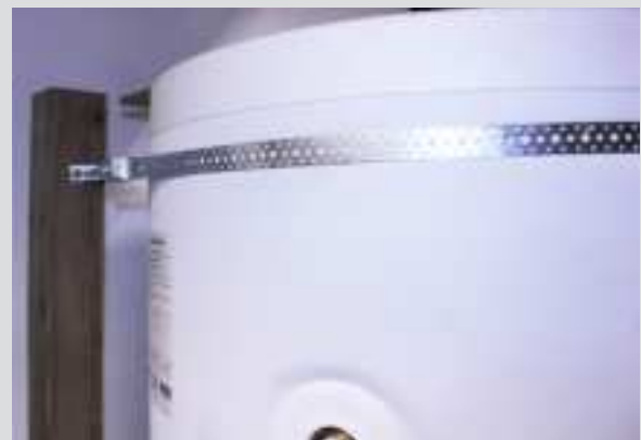
Seismic restraint needs to be determined by a calculation specific to the installation, as per NZS 4219.
