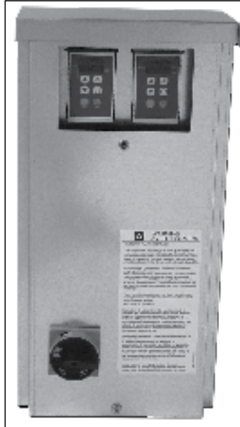
FIGURE 16.5.5 VFD KEYPADS IN EBOX
