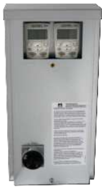
FIGURE 16.5.1 VFD KEYPADS IN EBOX
