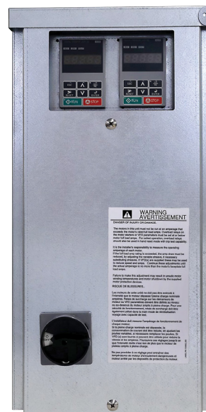
FIGURE 16.5.9 VFD KEYPADS IN EBOX
