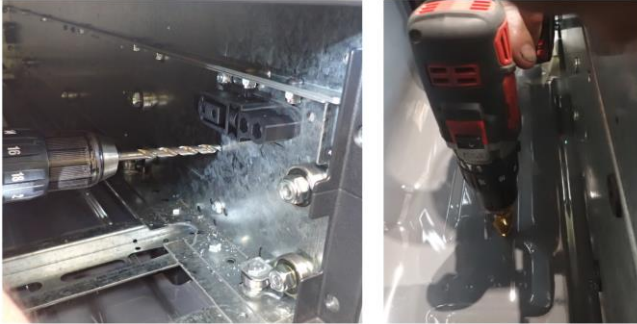
Drill pilot drilled holes to specified diameters
