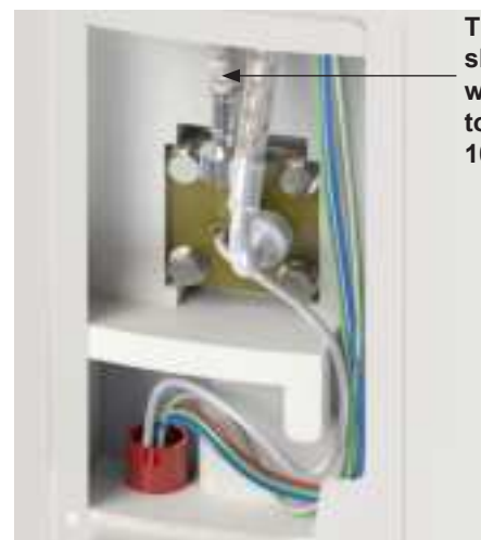
Heat pump hoses connected in the cylinder. Ensure there are NO KINKS in the hoses. Kinks can reduce the flow and cause a T1 fault.
