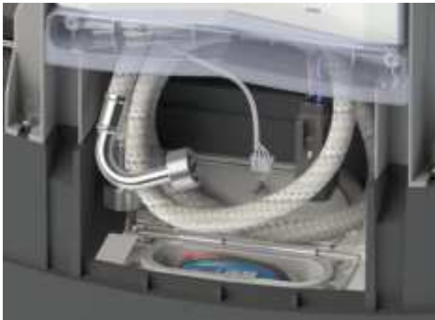
Heat pump hoses and electrical connections ready for connection to cylinder.
