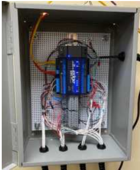
BASyC® Controls® Cabinet - includes capability for 2 loops (temp. zones) and up to 4 Mixing Valves.
