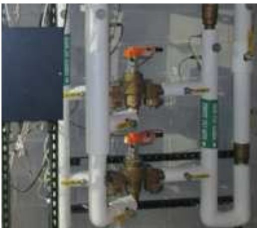
BASyC® System with SFMMV Dual-Valve Supply Fixture installed and operational at Lake Forest Medical Center, Lake Forest, IL
