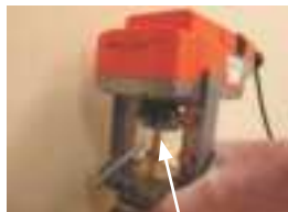
Make sure there is no gap between valve stem and actuator adapter—manually move, if necessary.
