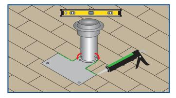
3. Adjust the top piece to make it straight and level, then bend the tabs over to secure it in place.
