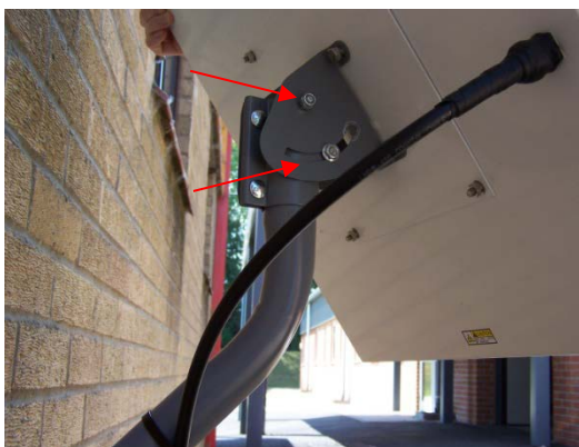
Figure 43: Adjusting elevation
