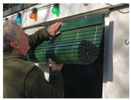
Optional for windows opening outwards. Fix 2 No. 35mm deep wooden batons on either side of the locking device to bring the blind forward and allow the window to slightly open.
