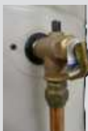
TPR position - top of cylinder
