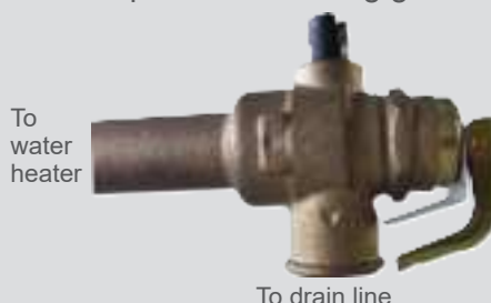
How to operate the easing gear
