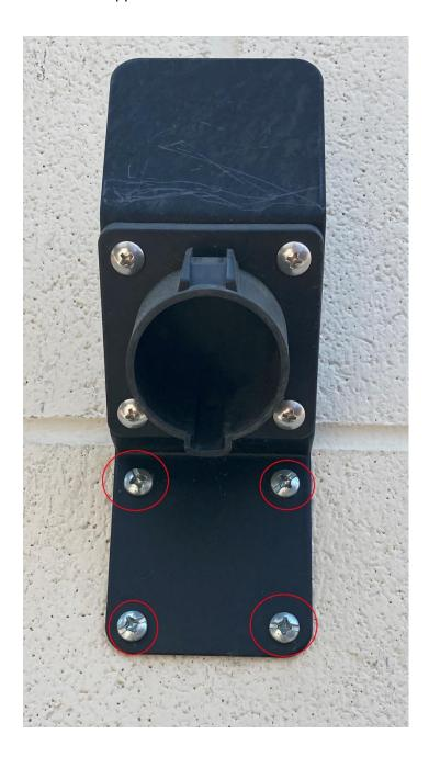
If the existing holster is broken but the holes are intact, simply remove the broken holster and replace with a new one.
