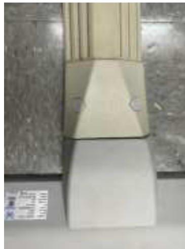
Figure 27: Where to Place Ground Pad Transition Piece
