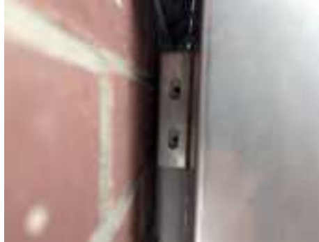
Figure 5: Wall Box Secured to Wall
