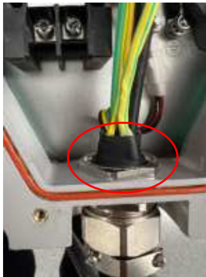
Figure 22: Nut Tightened Around Wires
