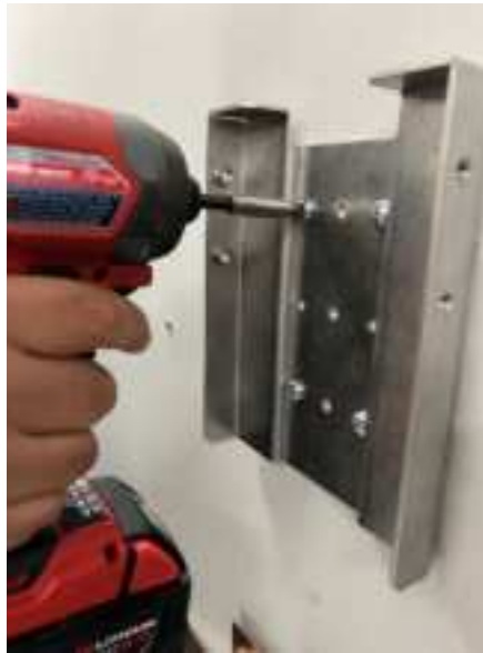
Figure 3: Driving screws into wall through bracket
