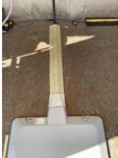
Figure 28: Ground Pad Assembled with Ground Conduit
