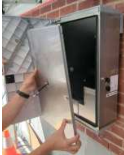
Figure 10: Removing the metal shield
