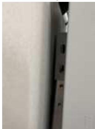
Figure 4: Wall Box Sliding onto Mounting Bracket
