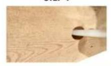
APPLY GENEROUS AMOUNT OF ADHESIVE INTO EACH HOLE PRIOR TO INSTALLATION THIS CREATES A PERMANENT BOND
