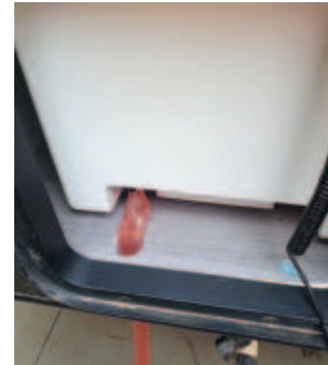
15 Slide vent hose through existing hole in floor
