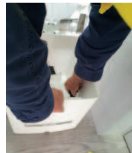
18 Place unit in position and screw to floor via reinforced points in the base
