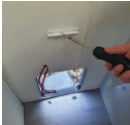
10 Unscrew the flush unit bracket from the wall
