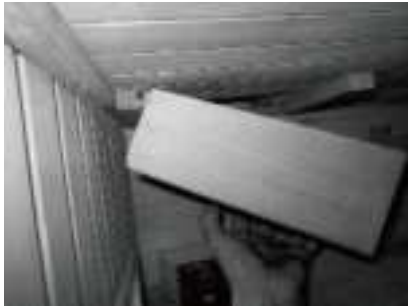
FIG-16 Installing the Radio Wood Housing
