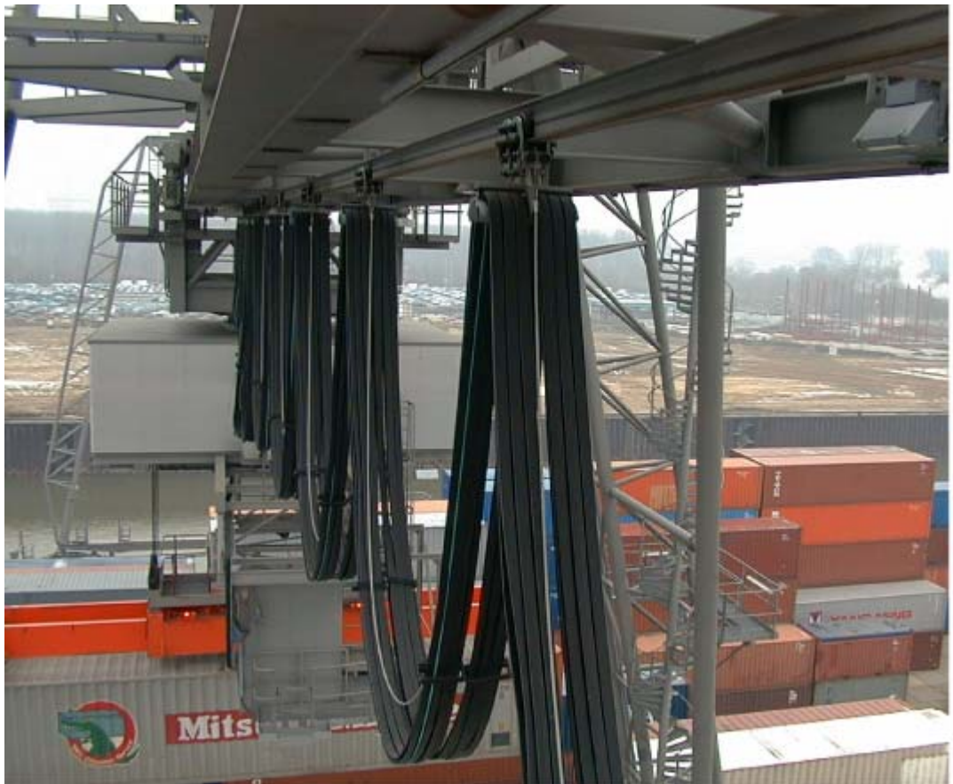
Figure 5-12 Example of the use of the PROFIBUS festoon cable
