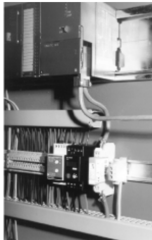
Figure B-3 Fine protection in the cubicle close to the first bus node
